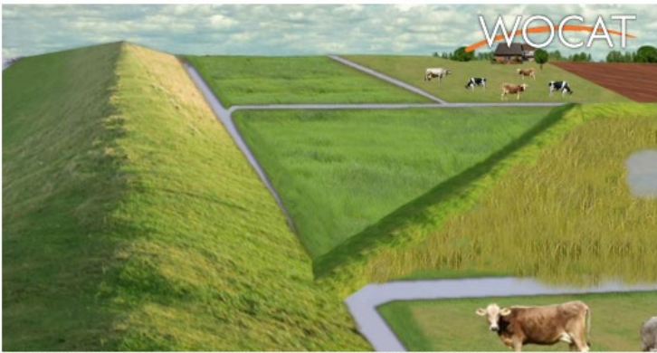
Water retention area at the primary sea wall with the delineation of the retention area and the land use as developed in a participatory process with local experts (Research project COMTESS)
