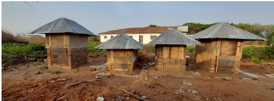
Figure 1. Low Energy Cool Barn
